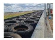
A new tyre wall has been placed trackside from post 5 thru to post 6 at The Bend. This will assist when cars hit the wall, and for those who have had the unfortunate experience of being on post 6 when a car has hit the wall. Hopefully this will see less damage and risk to drivers and officials.
